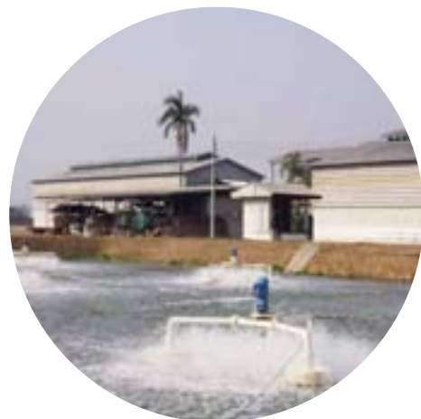
Aerobic wastewater treatment system
