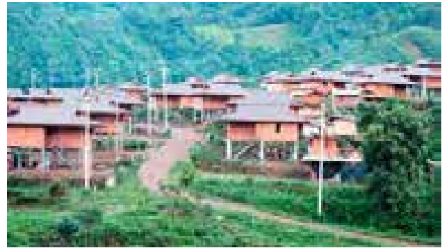
The "Baan Mun Kong" houses built for affected residents
