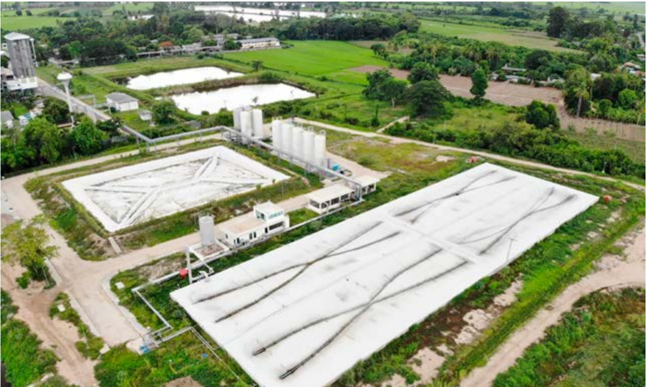
Biogas Plant Project in Nakhon Sawan Province
