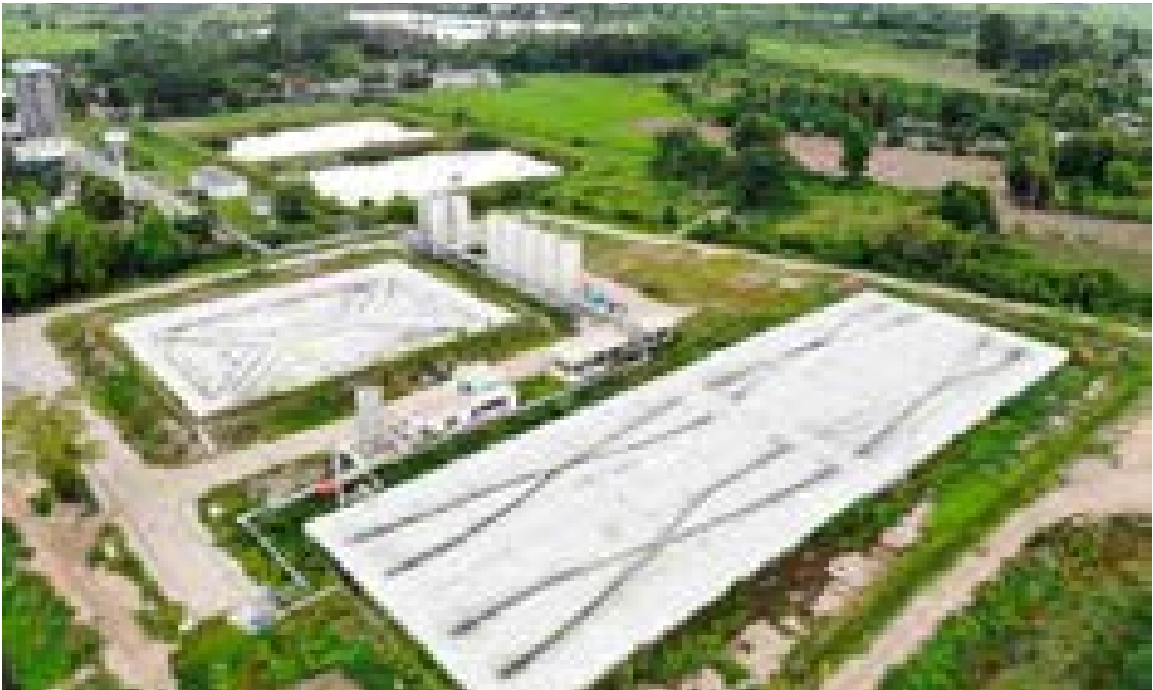
Biogas Plant Project in Nakhon Sawan Province
